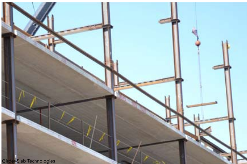
▲ Figure 5: Tree columns in place.
